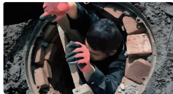
Sewage well dredging
