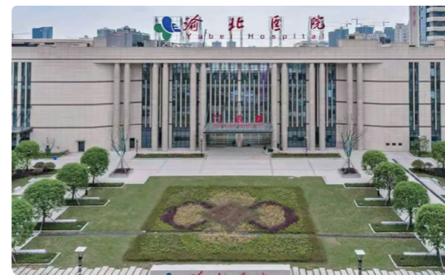
Ever Sunshine Services · Chongqing Yubei District People's Hospital Project
